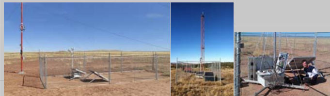
ATMOSCOPE installation at Meteor Crater site and the 30m anemometer tower
