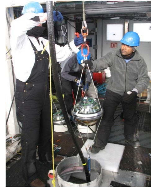
Installing an IceCube string
